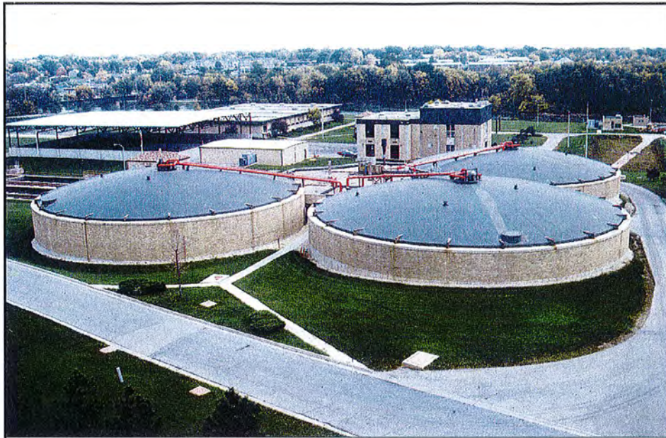
ANEROBIC DIGESTERS decompose organic matter.
