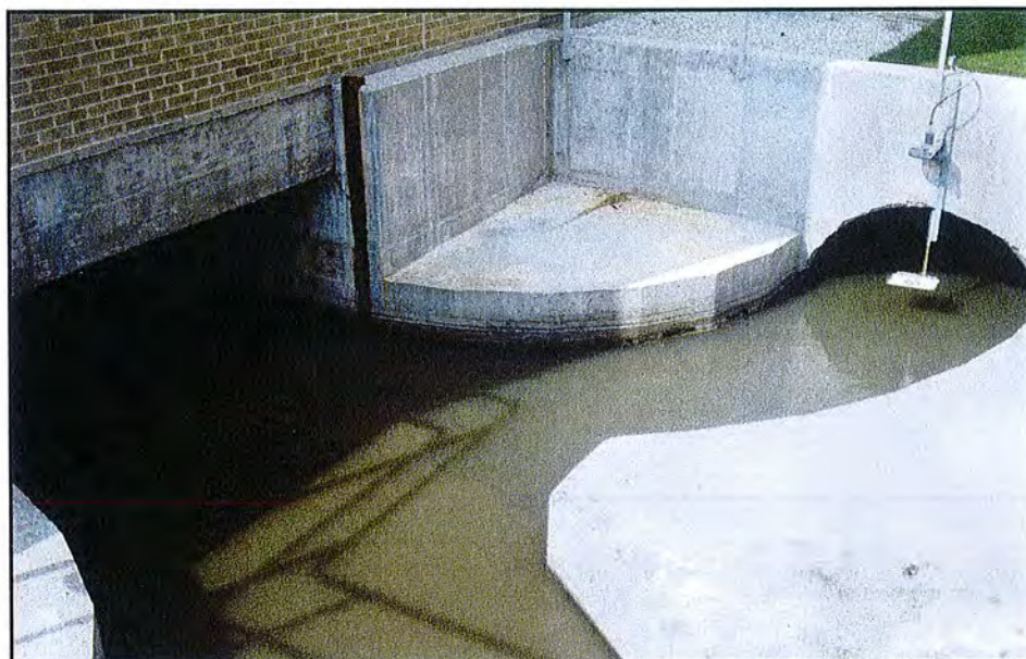
It all starts here. Raw Sewage
