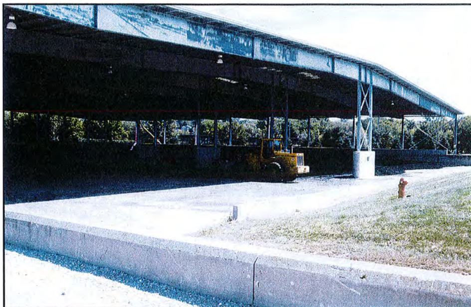
BIOSOLIDS are stored under a roof to keep them dry.
