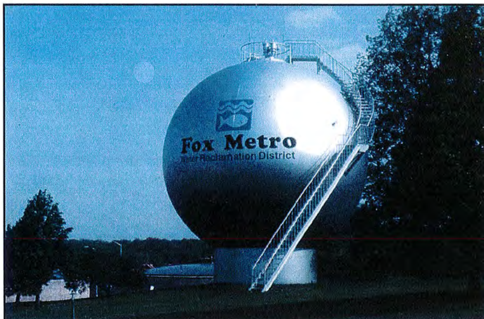
The methane gas produced is stored in a GAS SPHERE .
