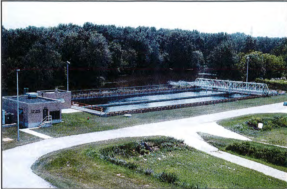
DISINFECTION TANKS help to sanitize the water.
